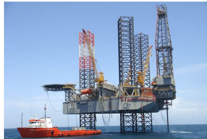
钻井平台 Drilling Platform
