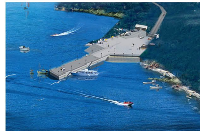
荣成市苏山岛陆岛交通码头 Rongcheng Sushan Island Traffic Quay
